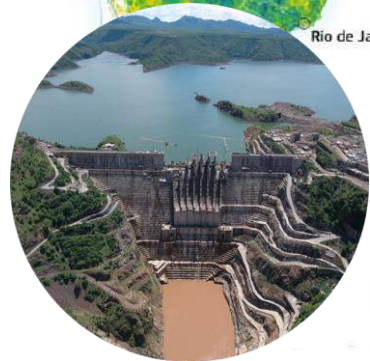
Gibe III Hydropower Plant on the Omo river in Ethiopia
